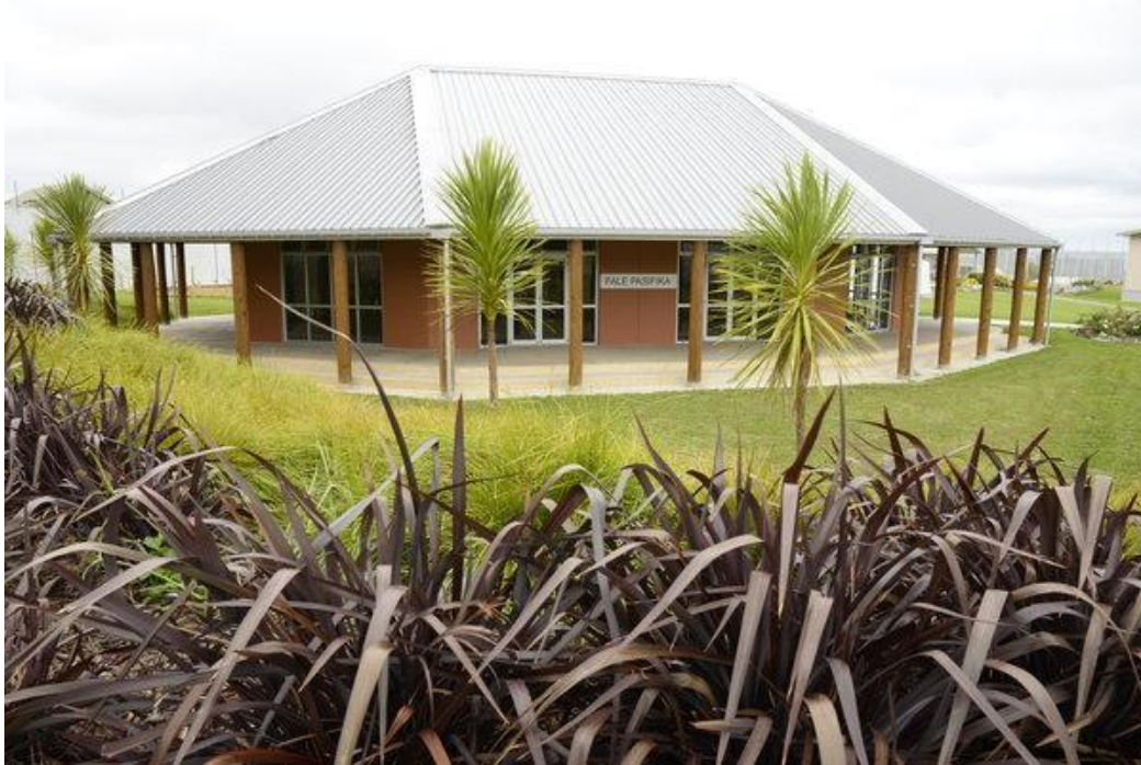
A Pacific communities cultural building, Fale Pasifika, at Auckland South Corrections Facility in New Zealand. Credit Serco New Zealand
