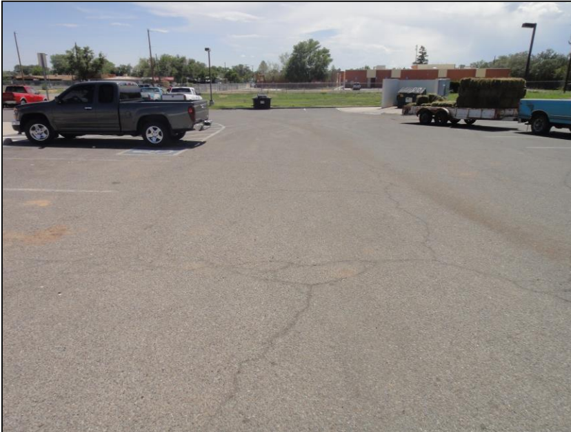
(Parking with no vegetation)
